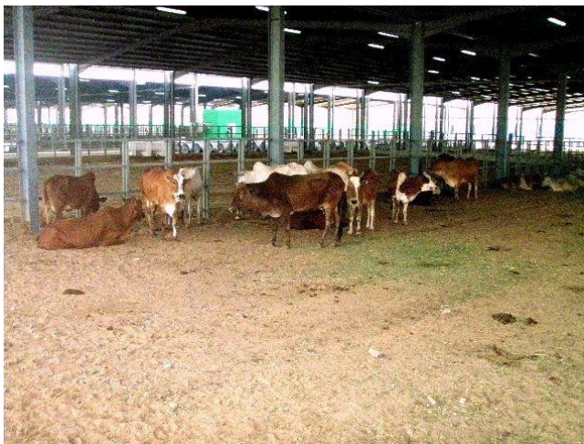
Figure 1. Open housing ease FMDV spreading
