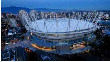
BC place Stadium For Football, Vancouver, Canada
