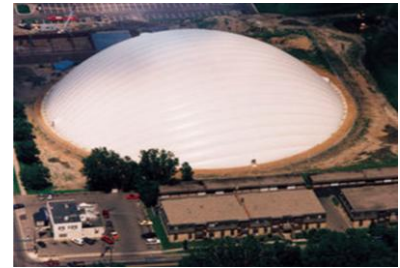
PVC coated polyester fabric (for air-supported structures) An air-supported structure utilizes an architectural fabric skin that is inflated by internal air pressure. Because there is no internal frame, the structure consists of only a fabric skin and a blower...
